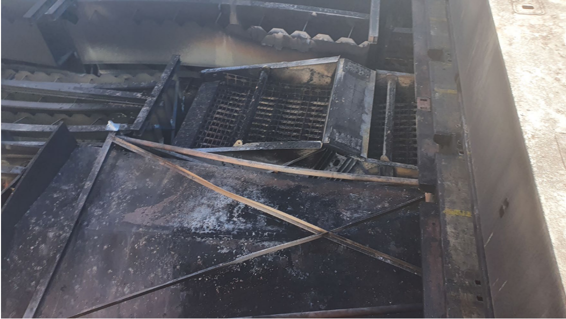
Figure 5: Burnt remains of the vibrating screen assembly
